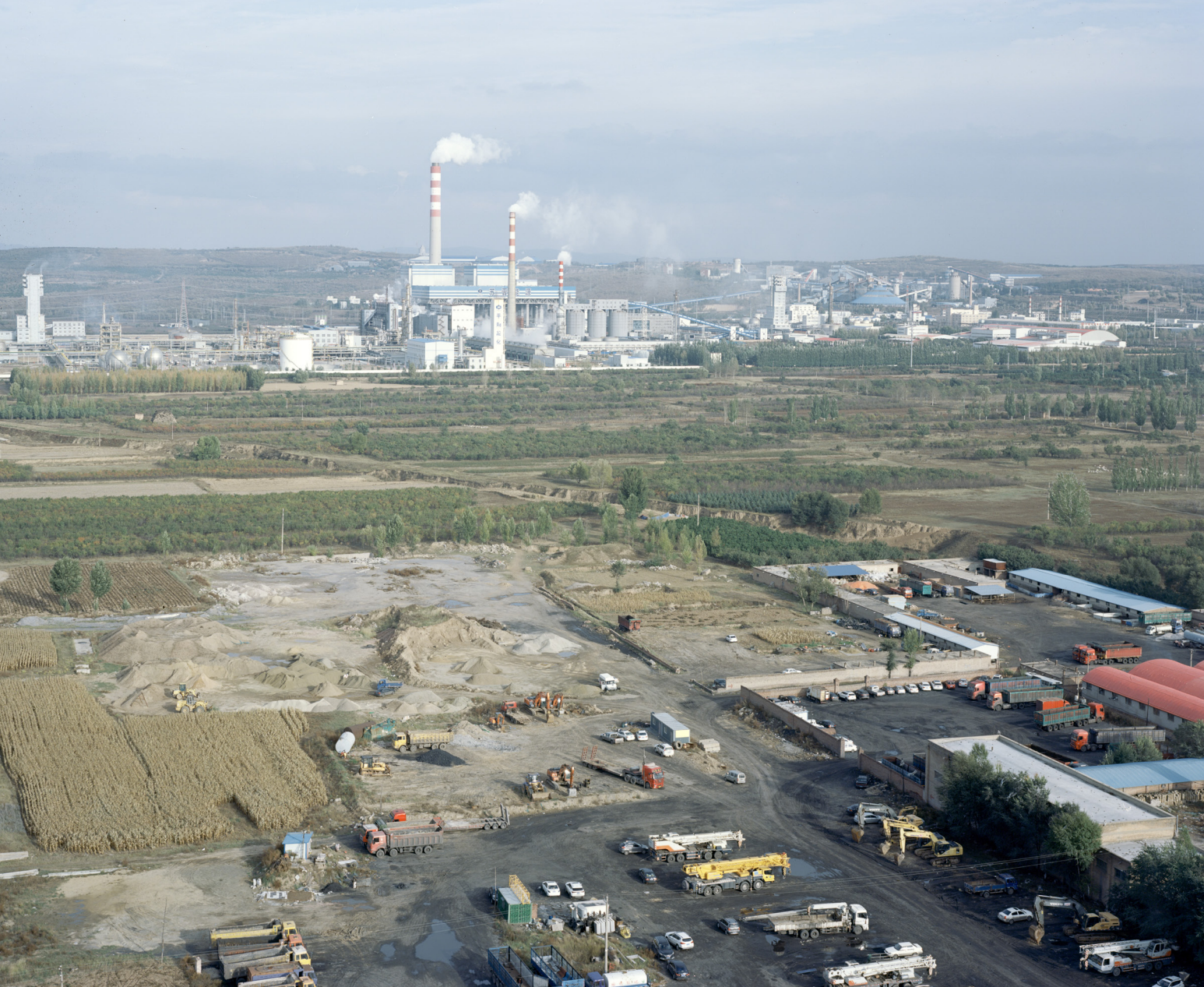
A gangue power plant. Coal gangue is also known as low-calorific coal, which is waste product from the mining and processing of coal. The satellite image of the same location and direction A tavern near the power plant
