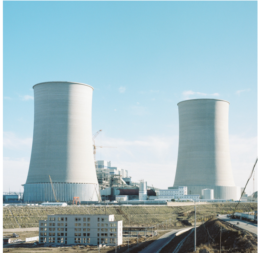
A coal-fired power station that is under construction, Shanxi Province
