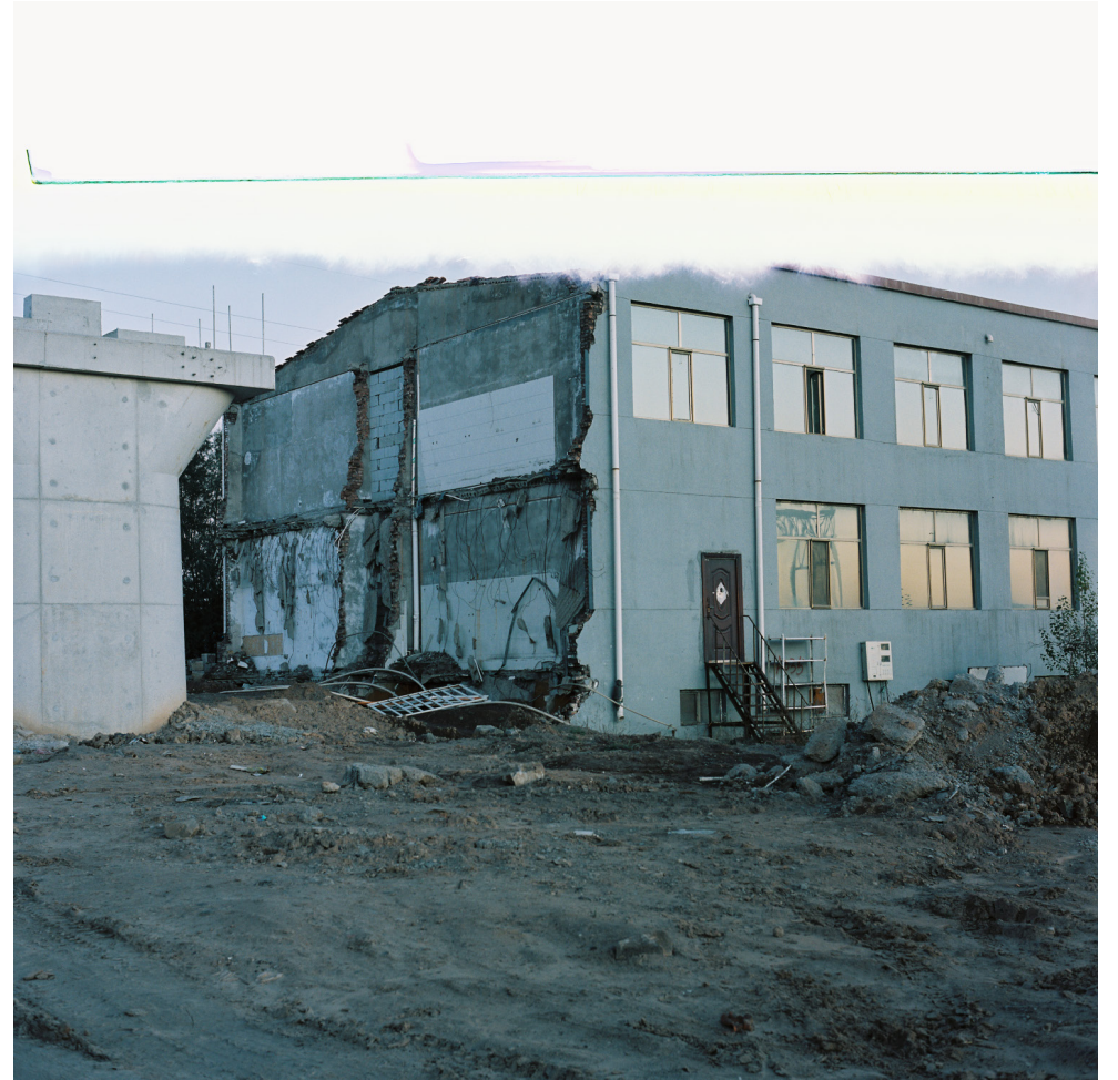
Dismantling for constructing, Shanxi Province
